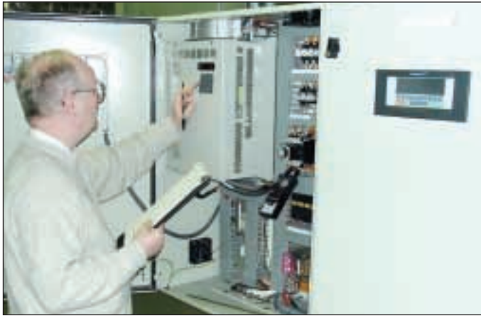
CAT Engineer measuring electrical energy consumption of air movement system
